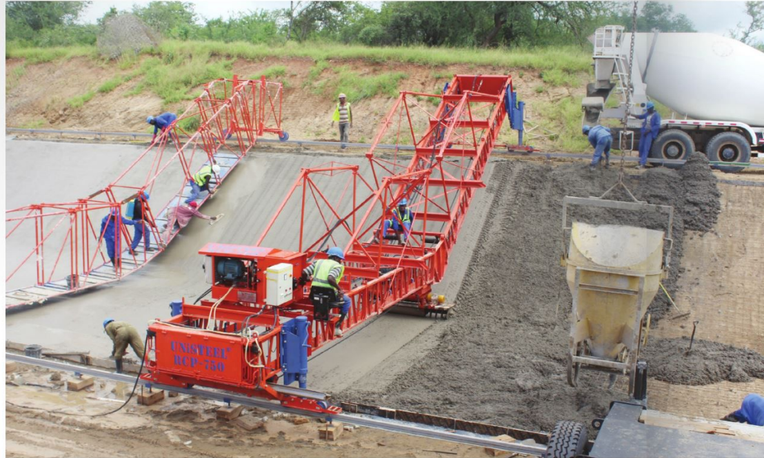
SVTP main canal under construction in Chikwawa
