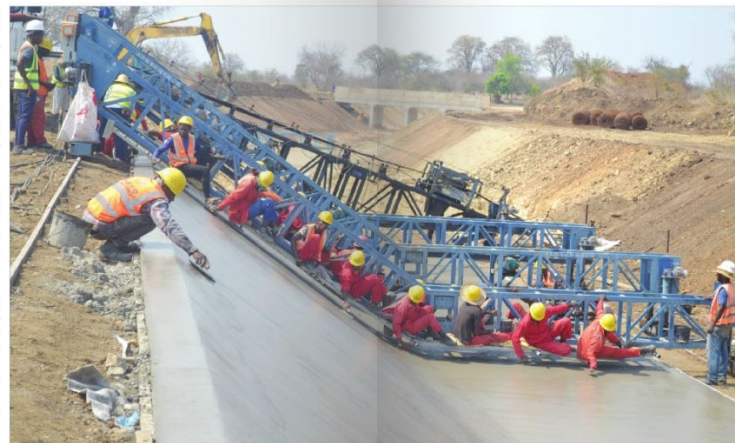
A section of the 118-kilometre irrigation canal under construction in Chikwawa
