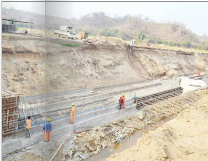
LEFELINE—The 1.18-Km Chikwawa-Bangula irrigation canal under construction
