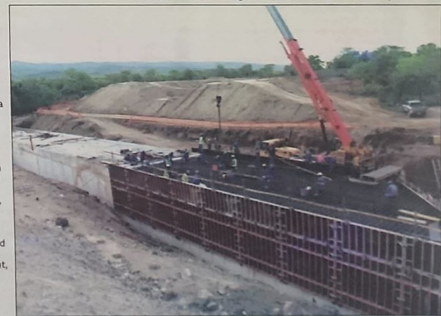
PROGRAMME ACTIVITIES—Works in progress on the Shire Valley Transformation Project
