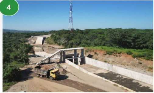
Picture 4: Completed 160 metres long siphon 1 connected to 396 metres long rectangular canal
