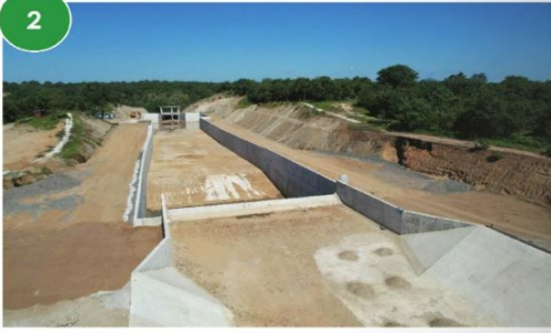
Picture 2: Completed 220 metres long tiger fish barrier
