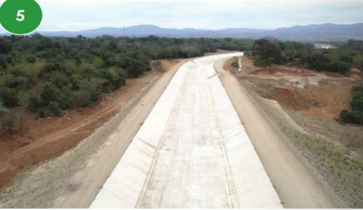
Picture 5: Part of the completed main canal
