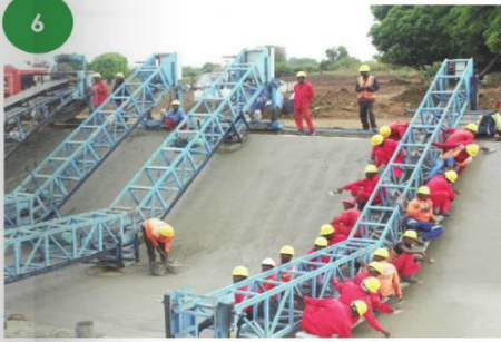
Picture 6: Canal alignment in progress in Chikwawa
