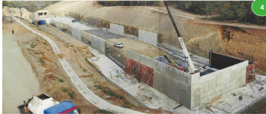
Pictures 1-6 provide some pictorial highlights on some major works taking place at the SVTP construction site in Chikwawa currently. Picture 1: Construction of 160 metre long Siphon 2 in progress, Picture 2: Part of the cleared canal route, Picture 3: Part of the 4.09kms concrete paved section of the canal, Picture 4: The 200 metre long tiger fish barrier structure under construction, Picture 5: One of the three completed bridges on the canal
