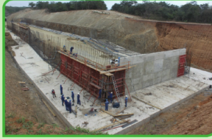
tiger fish barrier structure under construction
