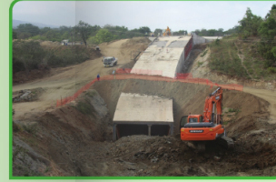
Siphon 2 under construction
