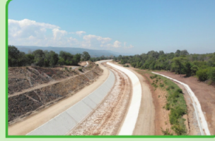
Part of the 409kms paved canal
