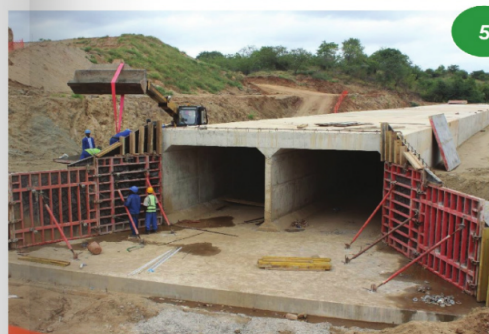
Pictures 1-6 provide some pictorial highlights on some major works taking place at the SVTP construction site in Chikwawa currently. Pictures 1-2: Some of the paved concrete sections of the canal, Picture 3: The flume within the Majete Wildlife Reserve, Picture 4: Construction of cut-off walls at the intake, Picture 5: One of the box culverts under construction as part of drainage works, Picture 6: Construction of Siphon 1 on the canal spanning 740 metres
