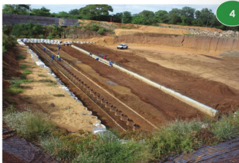
Pictures 1-6 provide some pictorial highlights on some major works taking place at the SVTP construction site in Chikwawa currently. Pictures 1-2: Some of the paved concrete sections of the canal, Picture 3: The flume within the Majete Wildlife Reserve, Picture 4: Construction of cut-off walls at the intake, Picture 5: One of the box culverts under construction as part of drainage works, Picture 6: Construction of Siphon 1 on the canal spanning 740 metres
