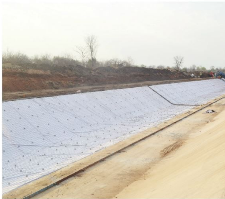
Part of the 118km canal under construction in the Shire Valley
