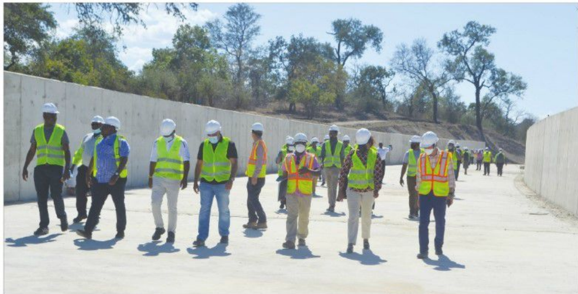
At some point, the canal is two metres high and five metres wide
