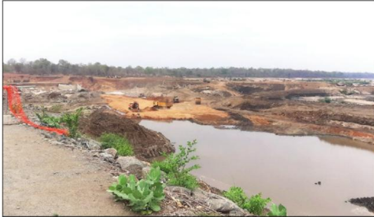
UNDER CONSTRUCTION—Kapichira water intake
