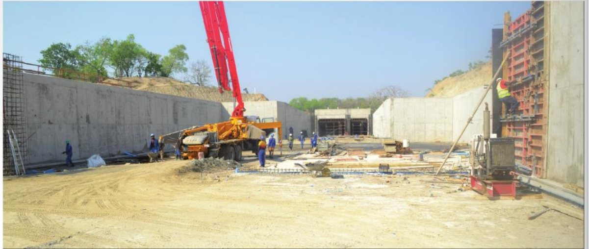
The SVTP's 118-km irrigation canal under construction
