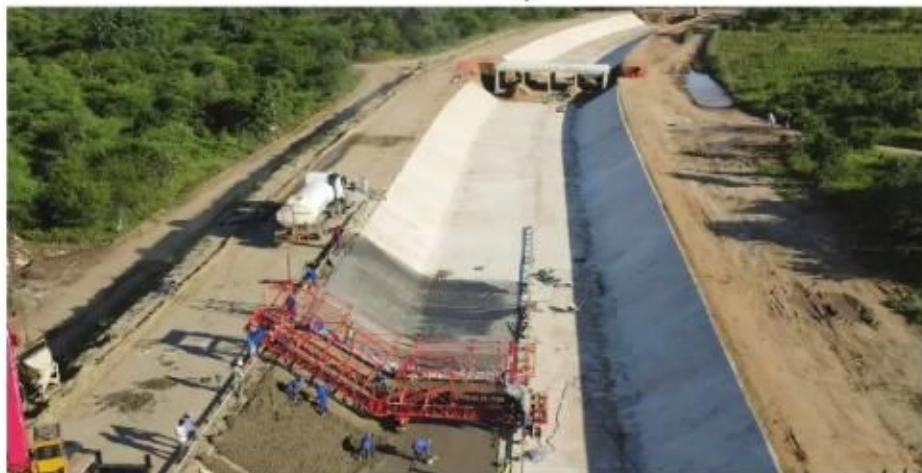
Part of the project currently under construction
