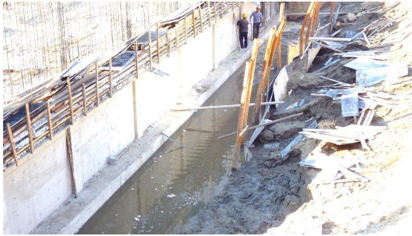
Figure 81: Working in damp condition around a pumping station (Source: BRLi, 2016 )
