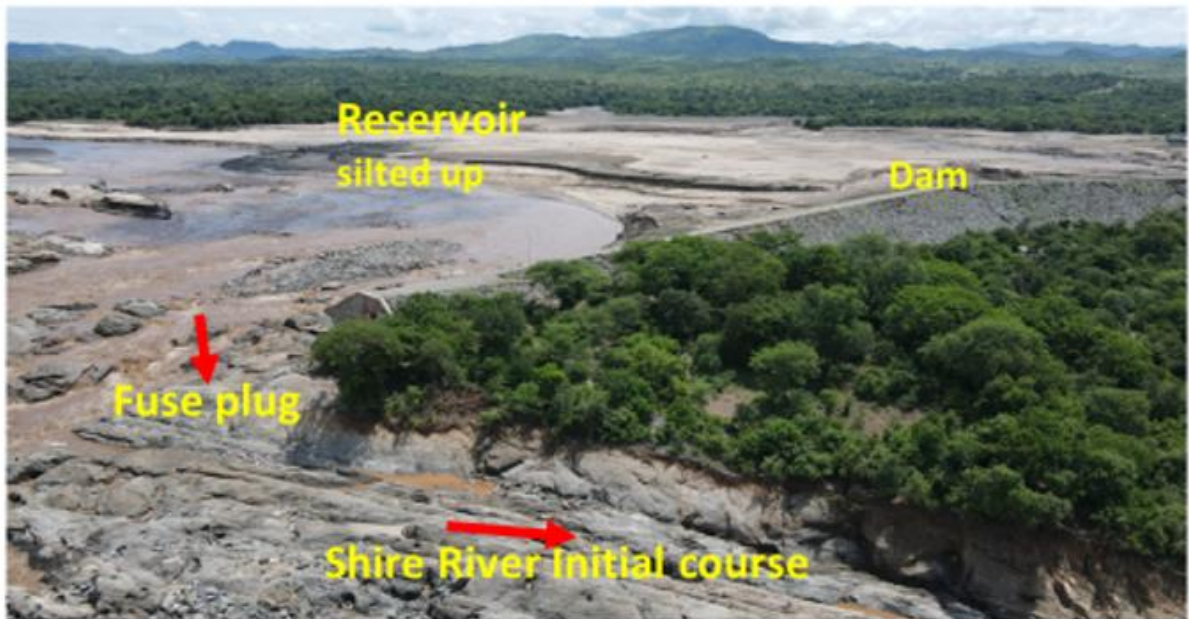
Figure 23: State of the Intake after Cyclone Ana
