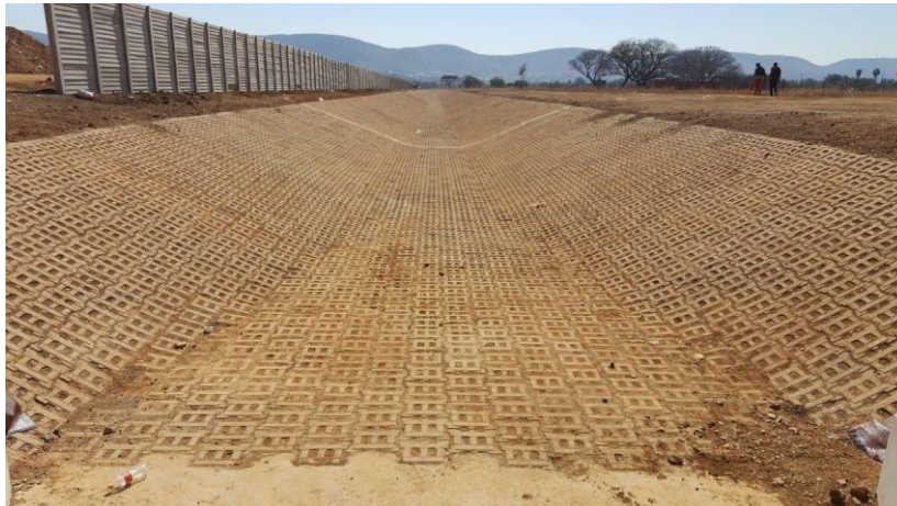
Figure 100: Armorflex (Source: ISG Infrastructure Specialist Group, 2016)
