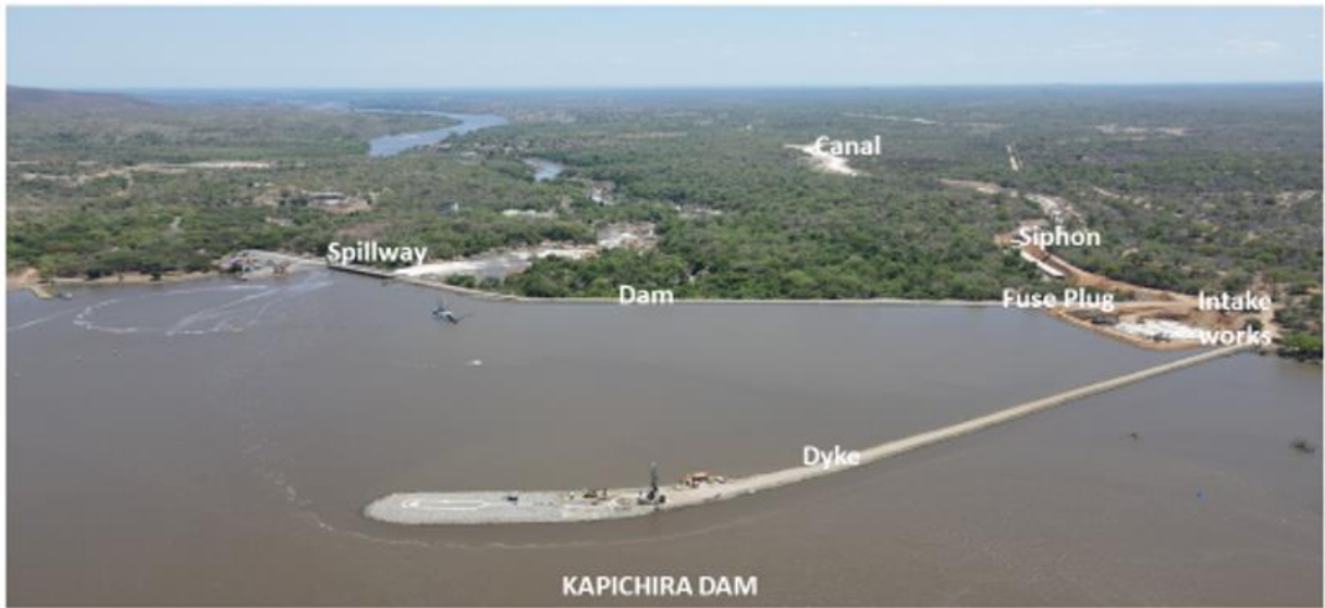
Figure 22: Original State of the Intake before Cyclone Ana
