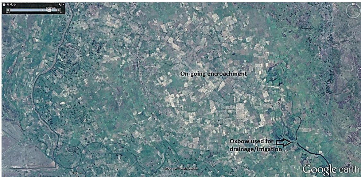
Figure 45: Ongoing encroachment of subsistence farmers following blockage of meander (2016)
