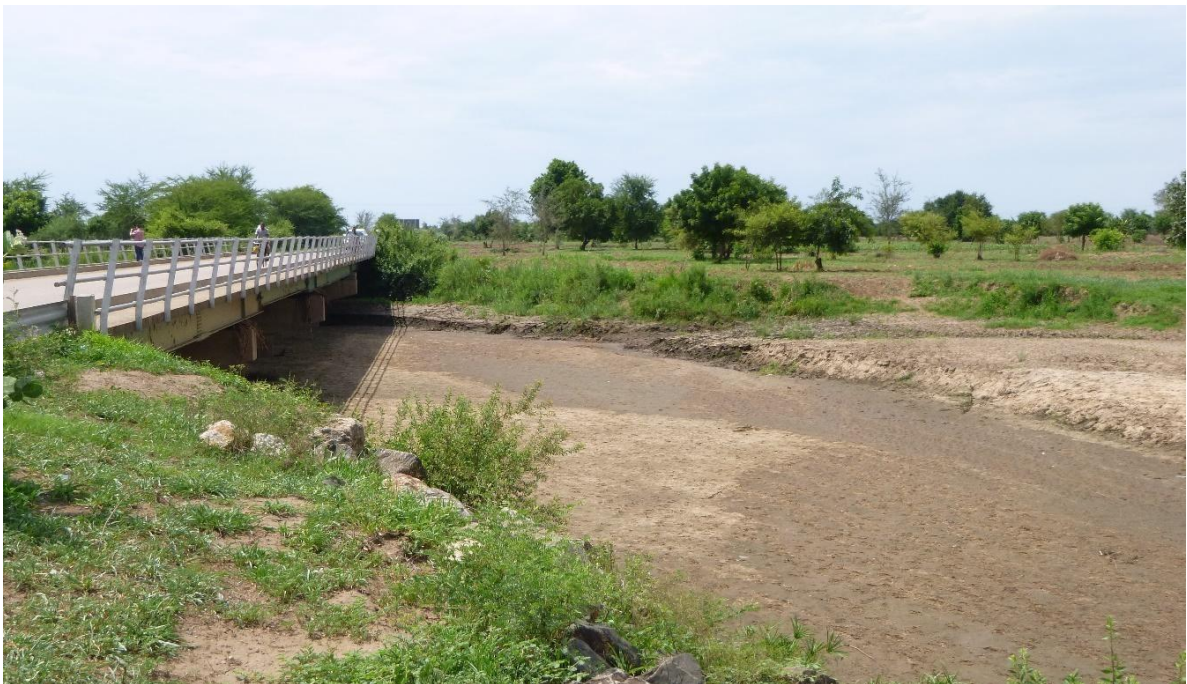
Figure 20: Mwanza River at the Bridge on the M1 Road
