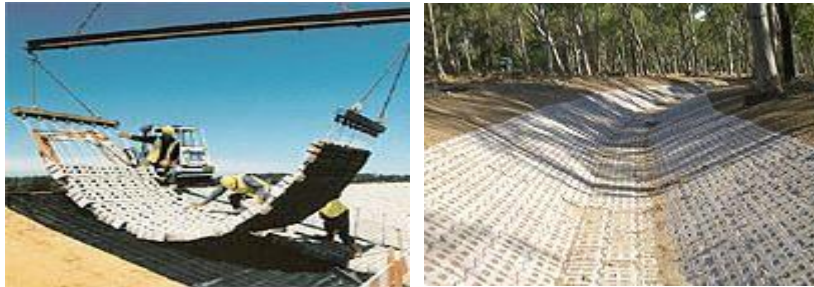
Figure 99: Prefabricated concrete mats (Armorflex®)
