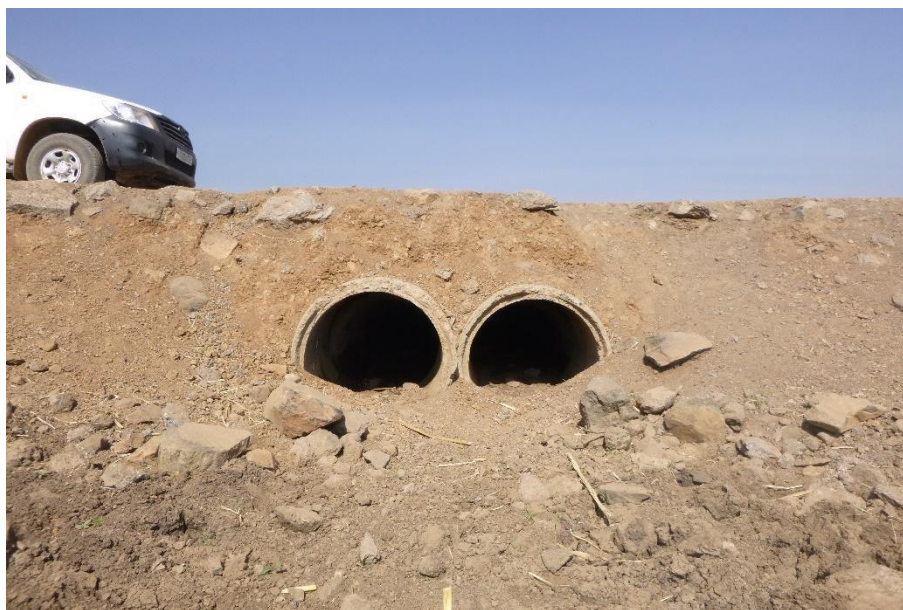
Figure 101: Inadequate culverts in an earth dike across a seasonal river (Source: BRLi, 2015)
