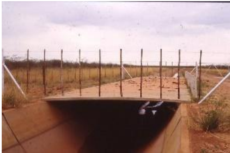
Figure 97: Overpass in Namibia (Source: Heyns, 2016 )
