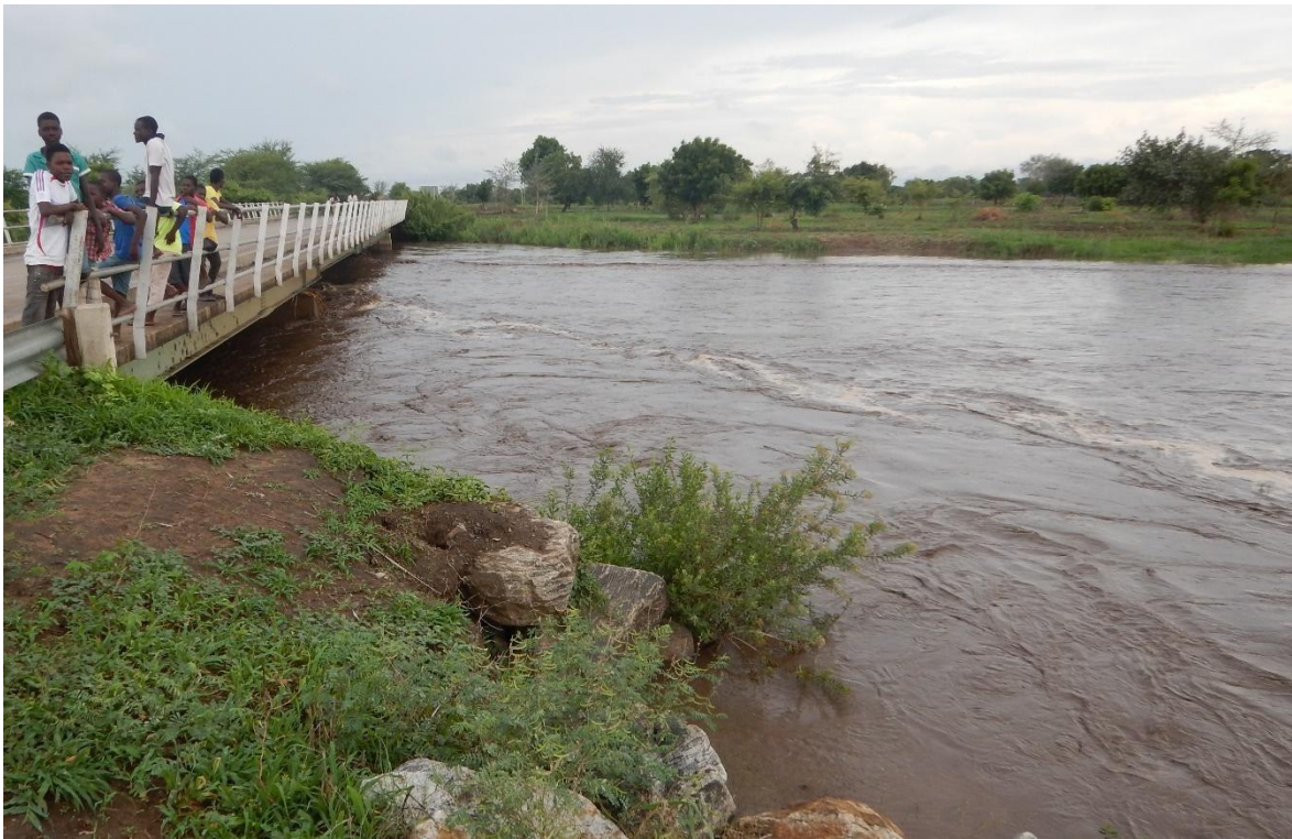
Figure 21: Mwanza River at the M1 Road during flooding
