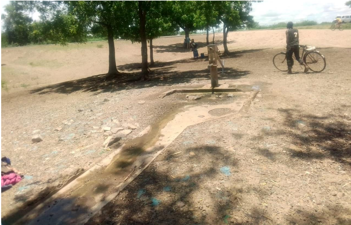
Figure 6-1: Picture of one of the affected boreholes
