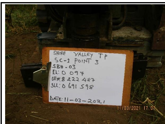
Drilling Rig Set Up for SBH-3
