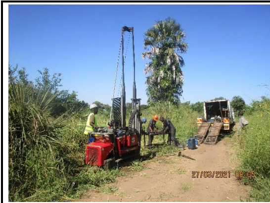
Drilling Rig Set Up for SBH-13
