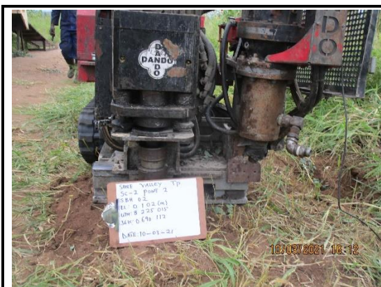
Drilling Rig Set Up for SBH-2
