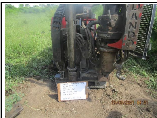
Drilling Rig Set Up for SBH-25
