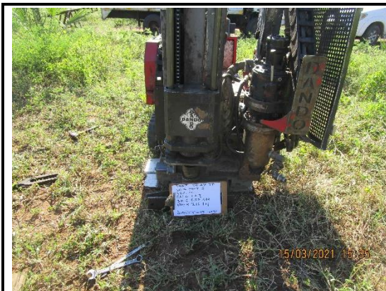
Drilling Rig Set Up for SBH-15
