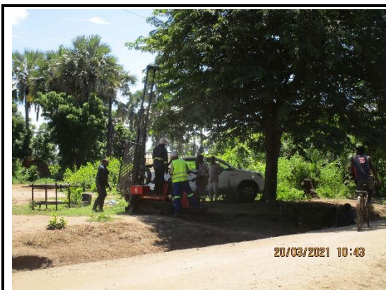
Drilling Rig Set Up for SBH-22
