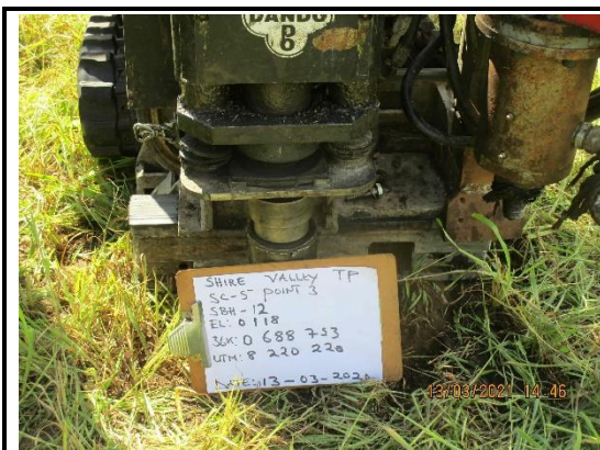
Drilling Rig Set Up for SBH-12
