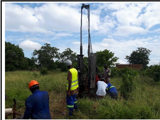
Drilling Rig Set Up for SBH-4
