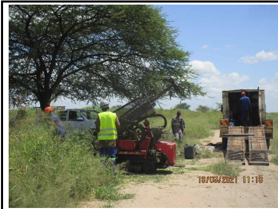
Drilling Rig Set Up for SBH-7
