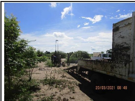
Drilling Rig Set Up for SBH-32
