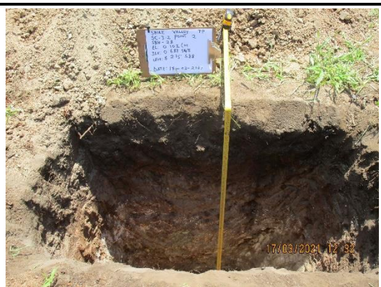
Digging Scene of SBH-28
