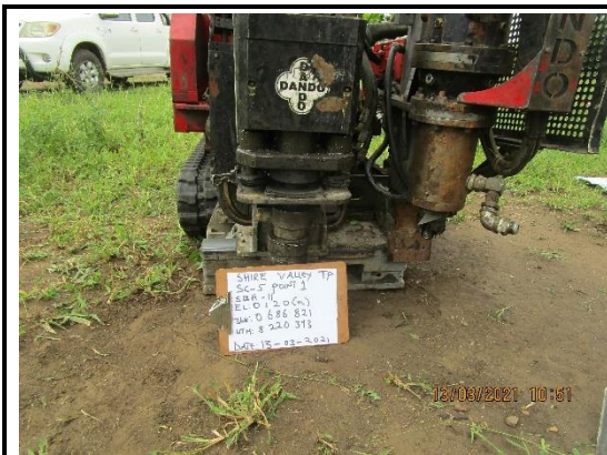
Drilling Rig Set Up for SBH-11
