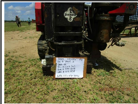
Drilling Rig Set Up for SBH-16
