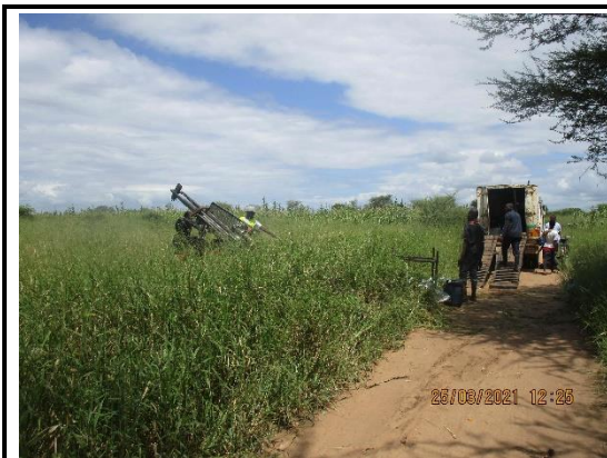
Drilling Rig Set Up for SBH-21
