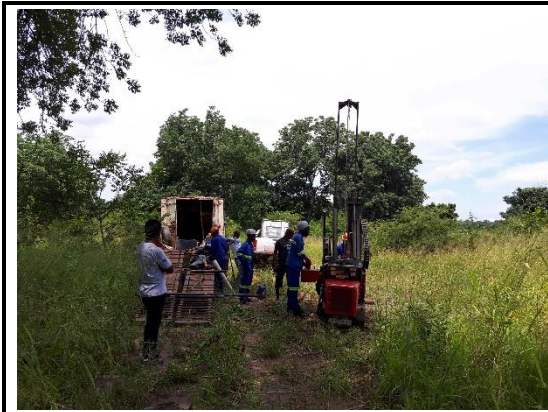
Drilling Rig Set Up for SBH-1
