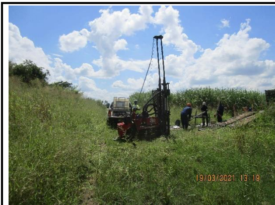
Drilling Rig Set Up for SBH-6
