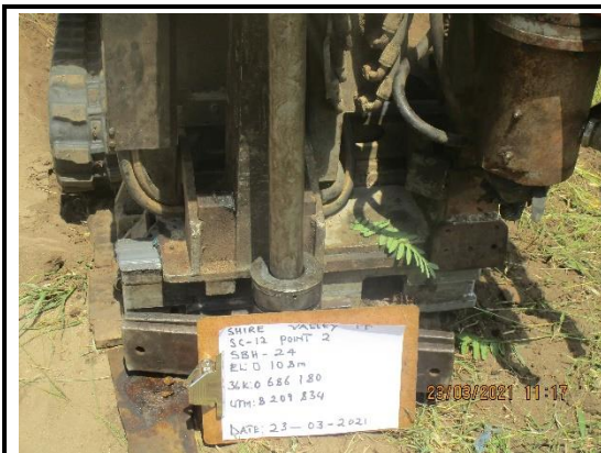
Drilling Rig Set Up for SBH-24
