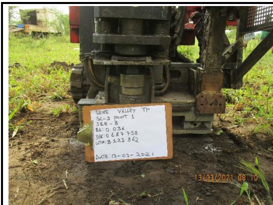
Drilling Rig Set Up for SBH-8
