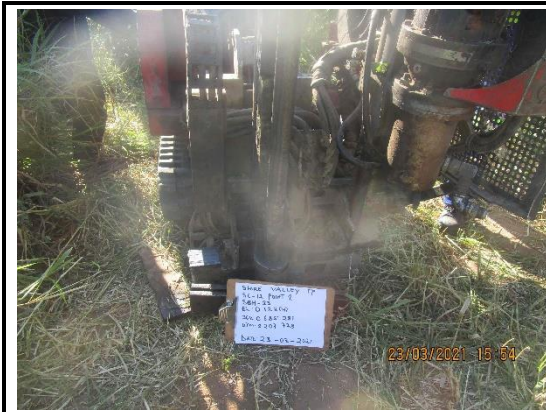
Drilling Rig Set Up for SBH-23
