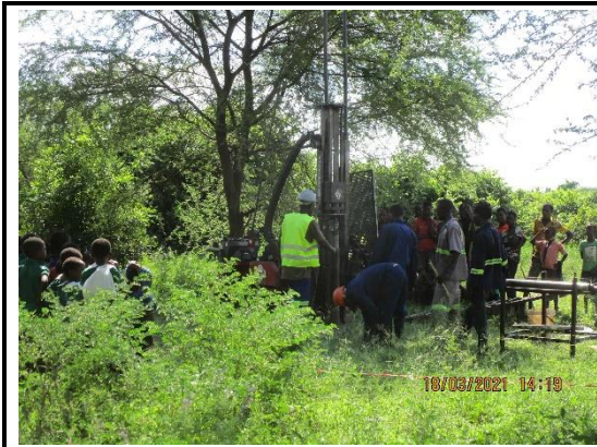
Drilling Rig Set Up for SBH-30
