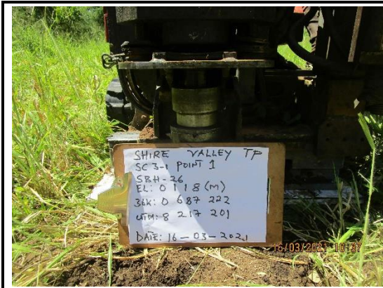
Drilling Rig Set Up for SBH-26
