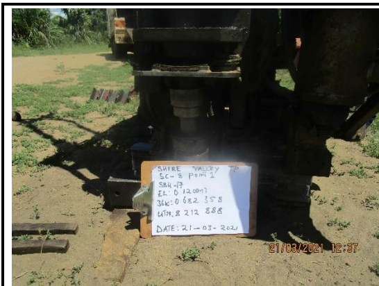
Drilling Rig Set Up for SBH-17
