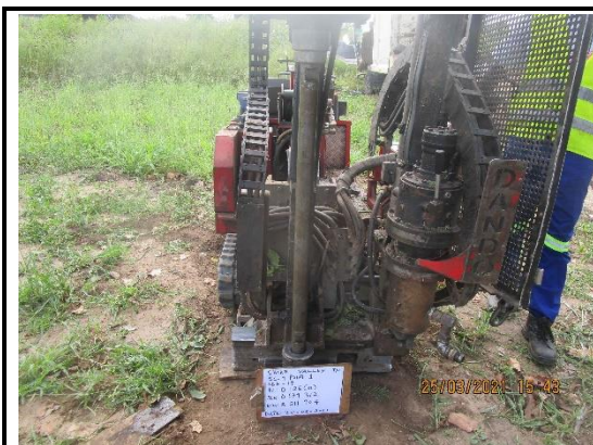
Drilling Rig Set Up for SBH-19
