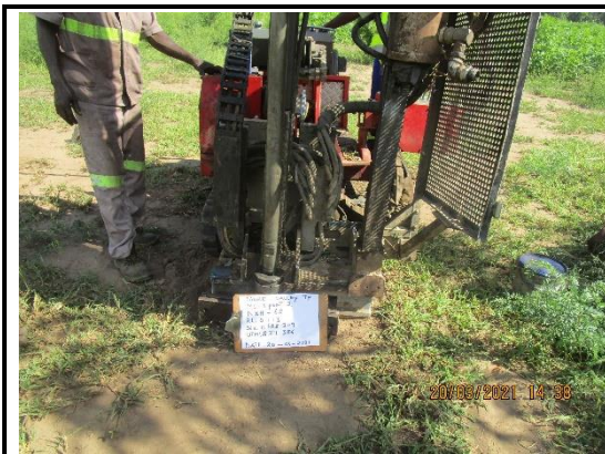
Drilling Rig Set Up of DBH-65
