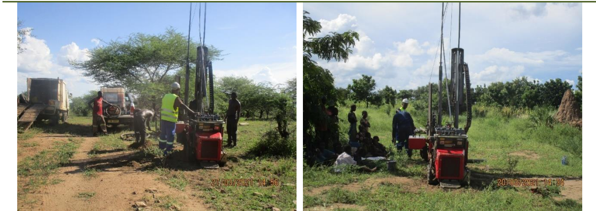
[Figure 1.7-1] Drilling of Boreholes
