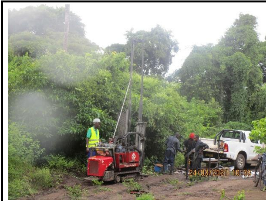
Drilling Rig Set Up for SBH-20
