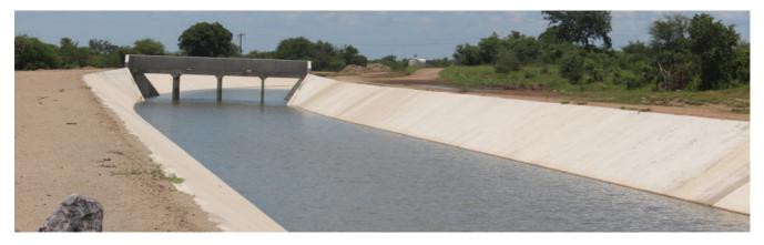
This is designed to convey a maximum of 50 cubic meters of water per second. However, the cross-section keeps on reducing in size with the subsequent withdrawal of water by secondary pipelines.
