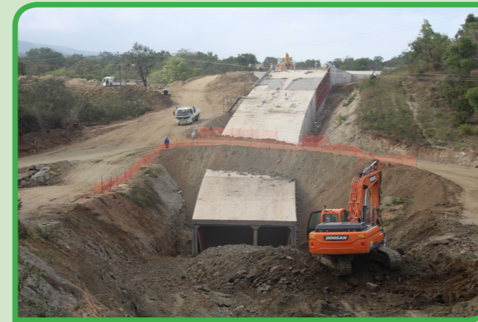
Siphon 2 under construction
