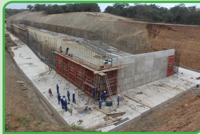
tiger fish barrier structure under construction
