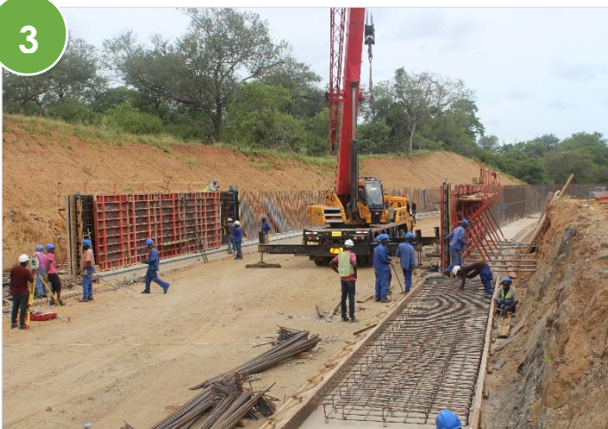
1: Construction of the cut-off wall at the intake
