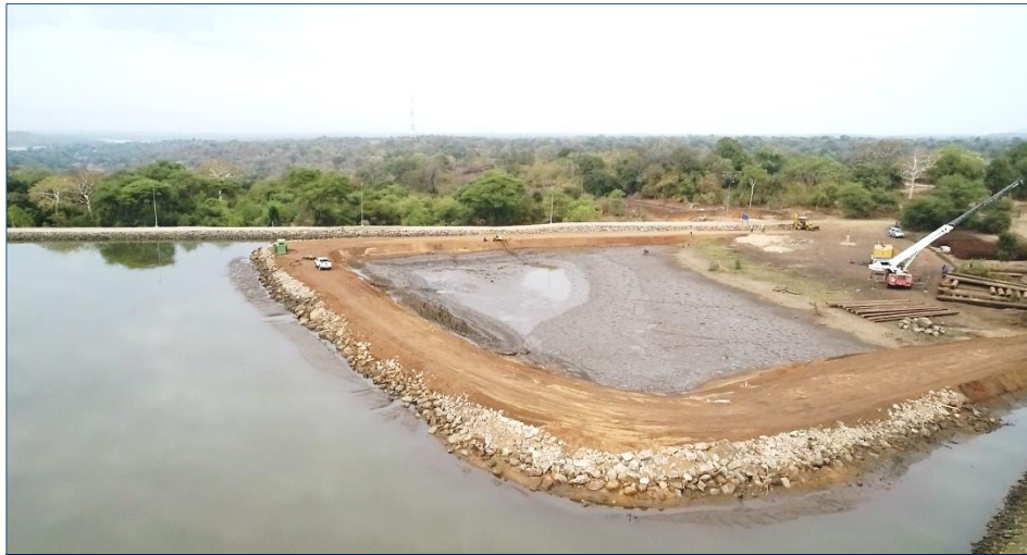
Draining water from the coffer dam
