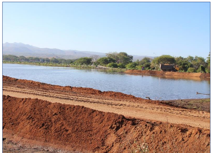
Coffer dam construction at the Intake
