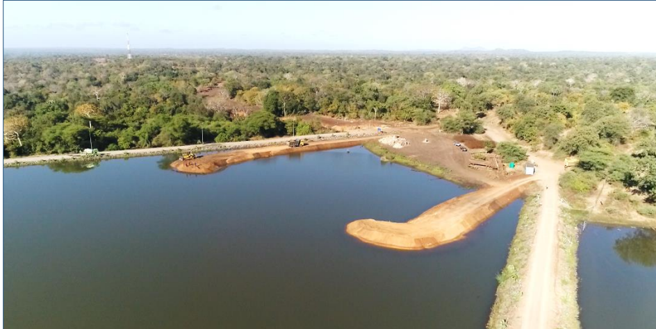
Construction of the coffer dam in progress
