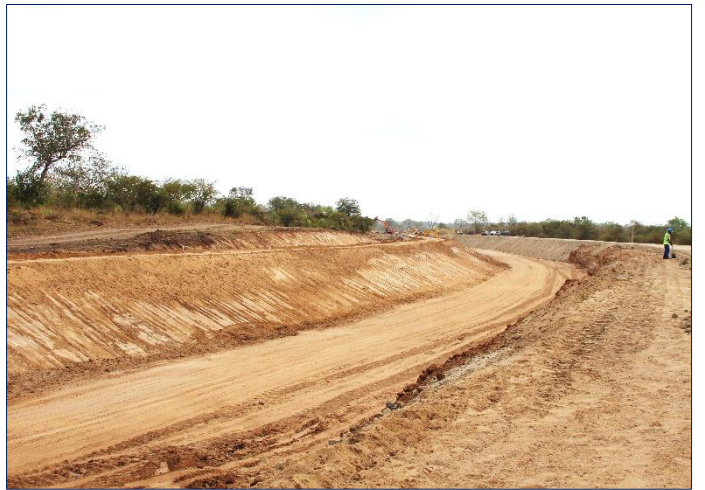
Coffer dam construction at the Intake
