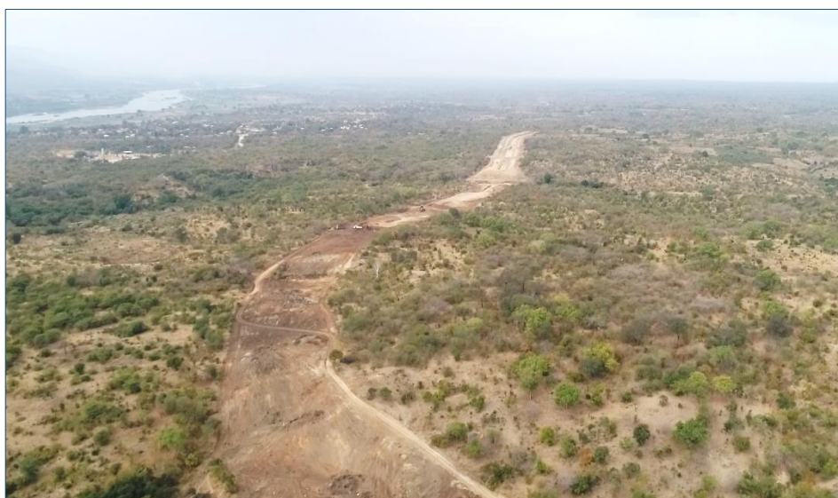
The cleared canal route
