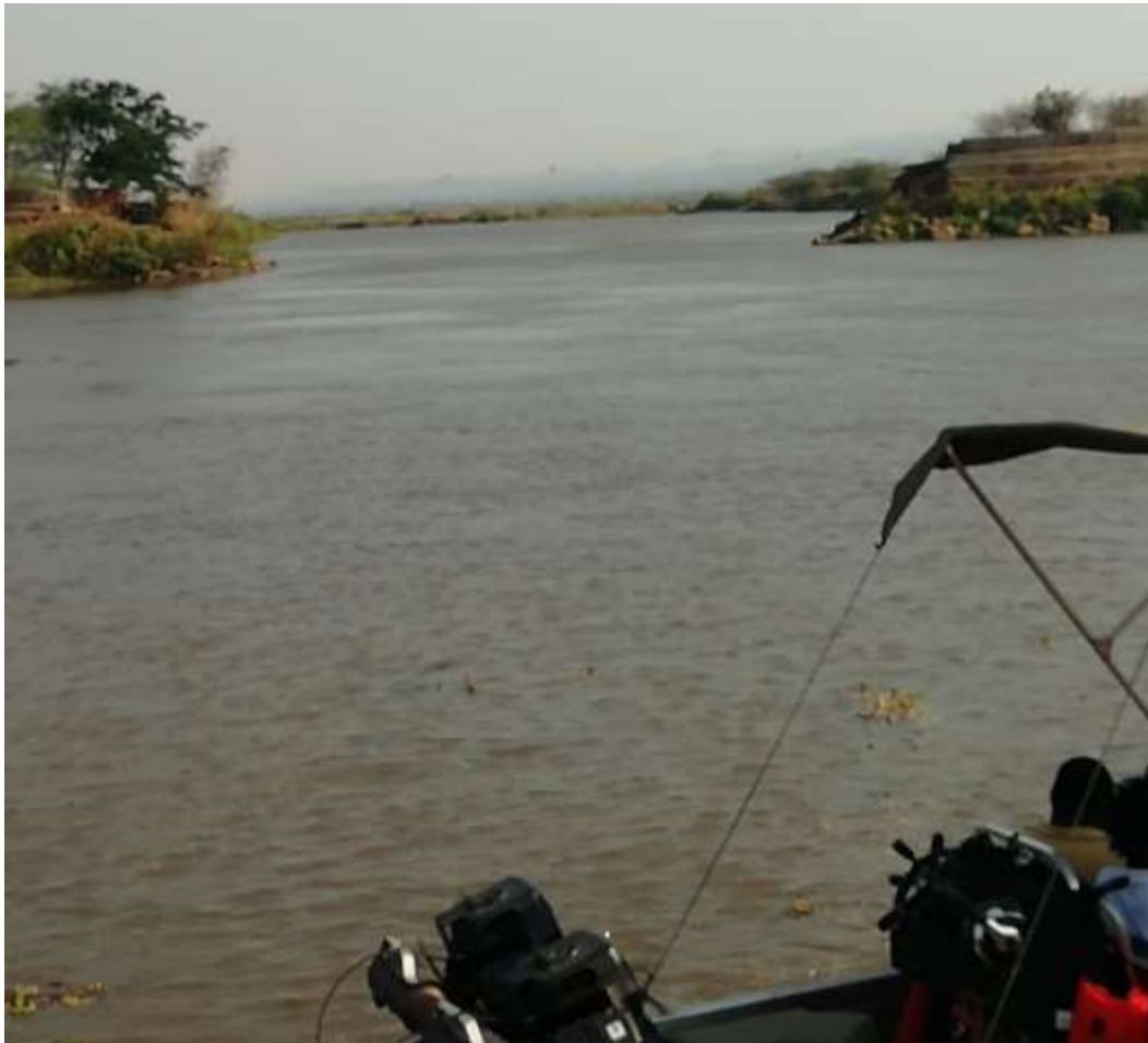
Figure 30: Washed away Rail Bridge across Shire River at Chiromo
