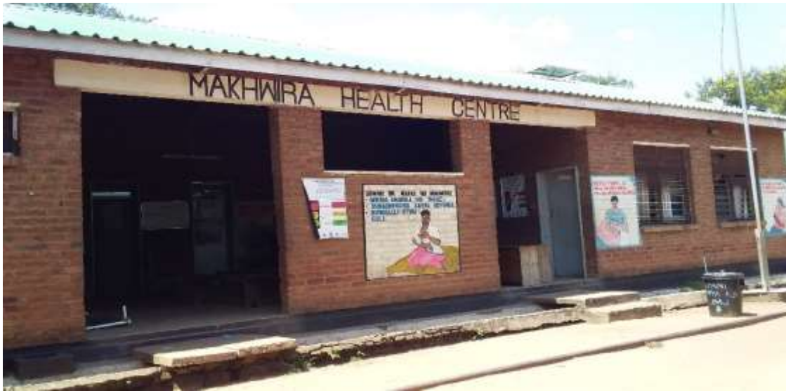
Figure 44 Makhwira Health Centre
