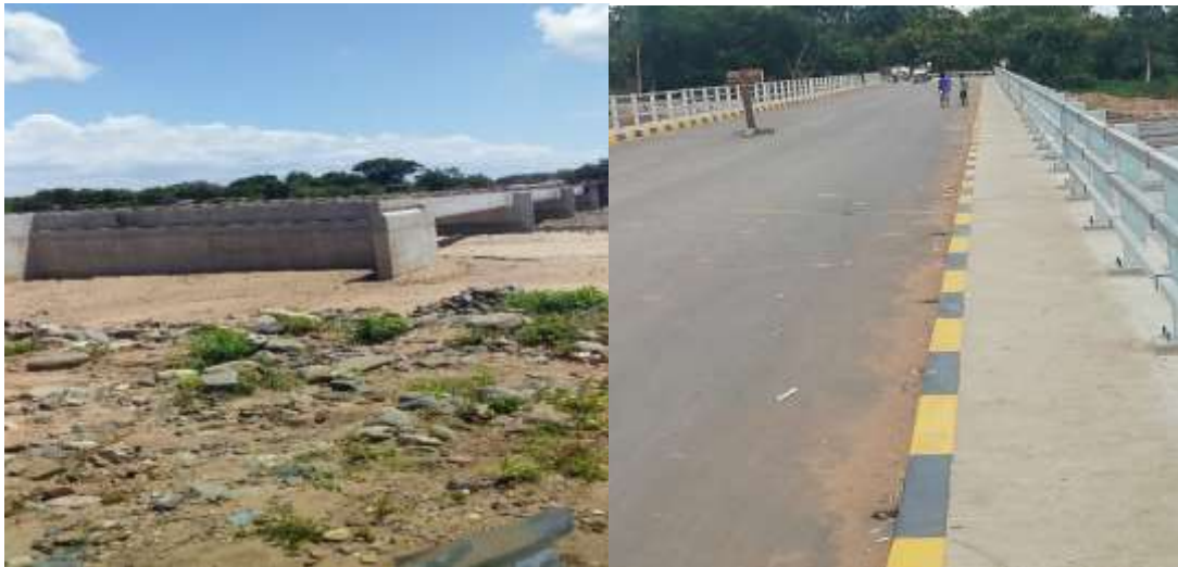
Figure 29: Livunzu and Chapananga Bridges
