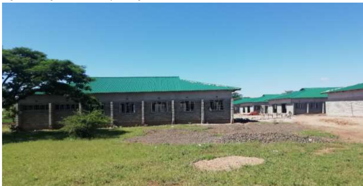
Figure 50: Ngabu Community College (under construction)
