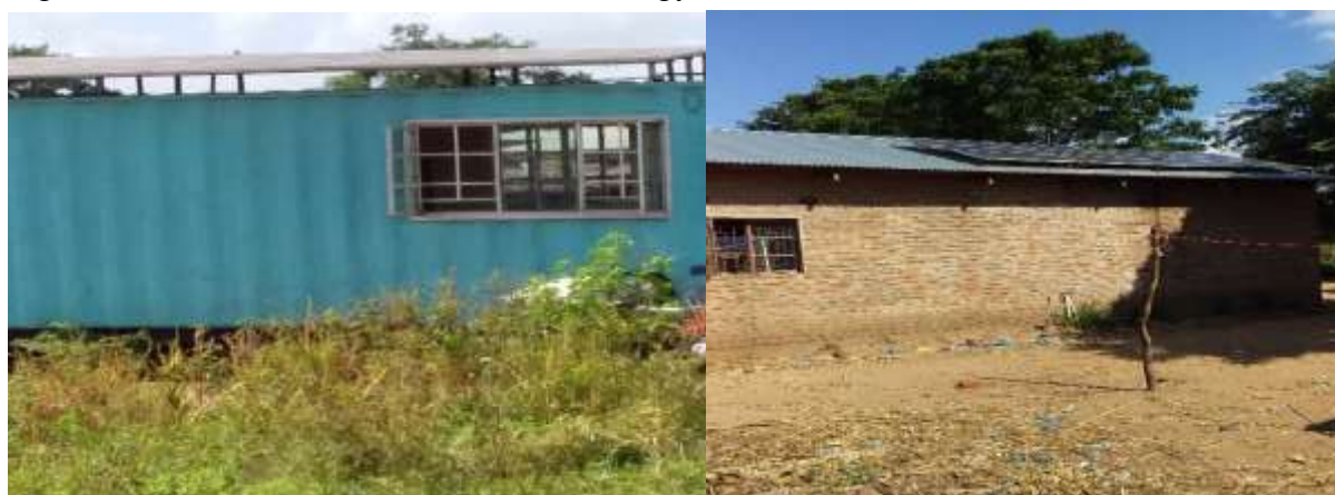
Figure 34: Thendo and Mandirade Solar Energy
