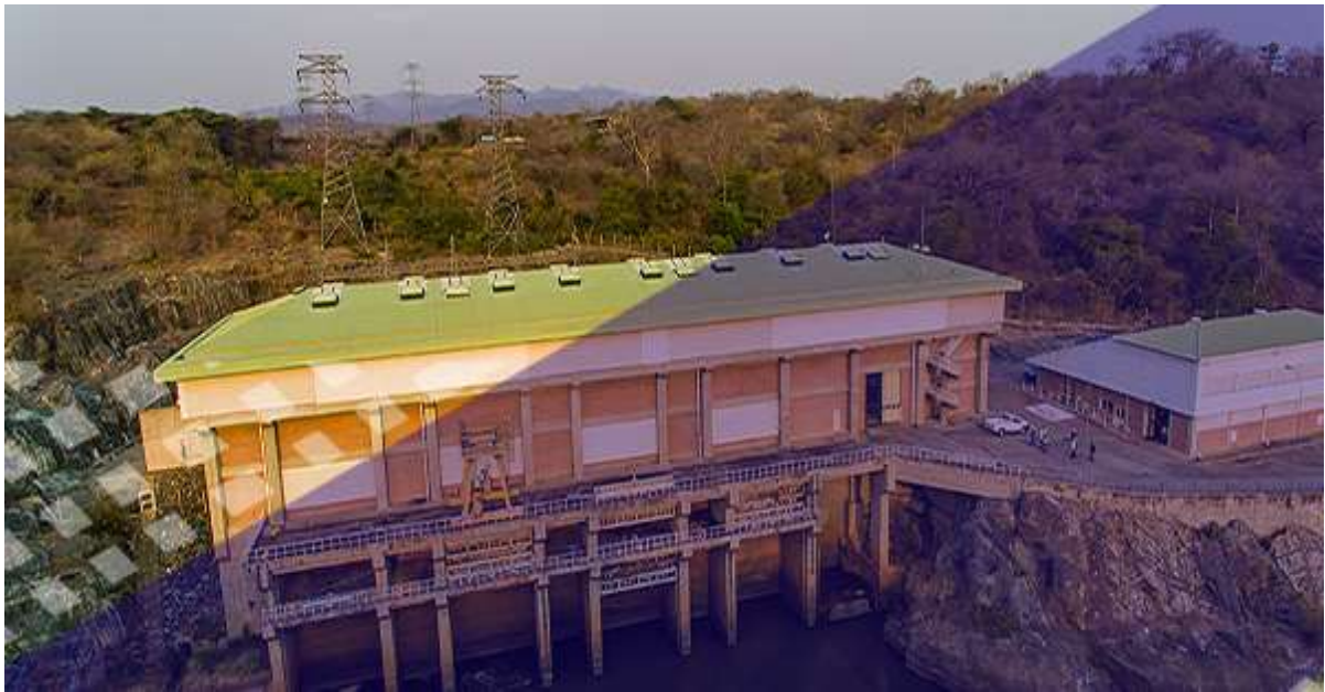
Figure 32: Kapichira Hydro Power Scheme
