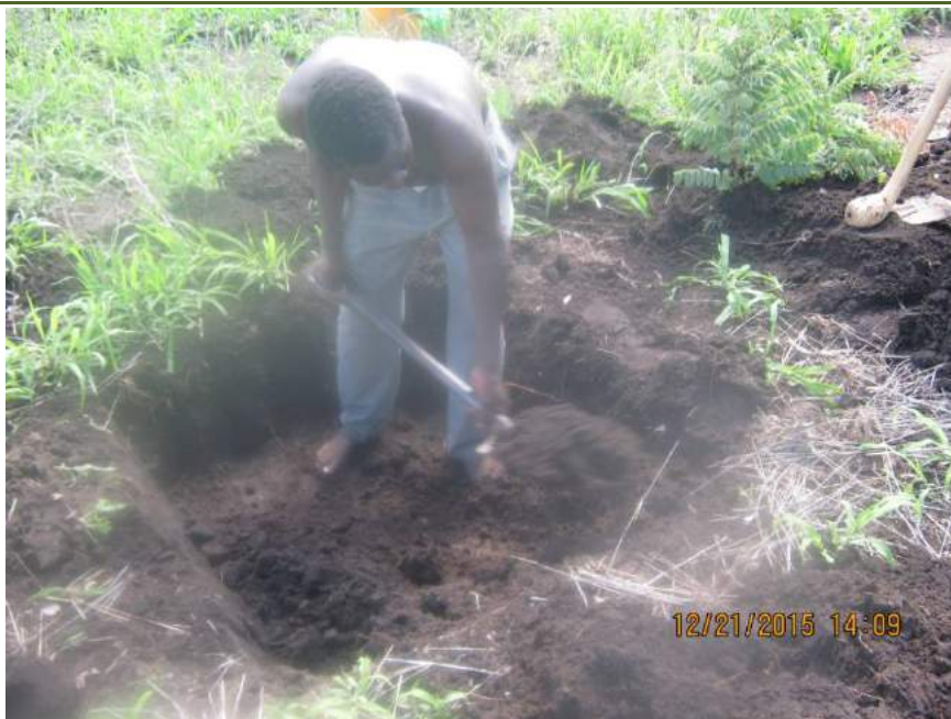
[Figure 2.3-4] Digging the Pit
