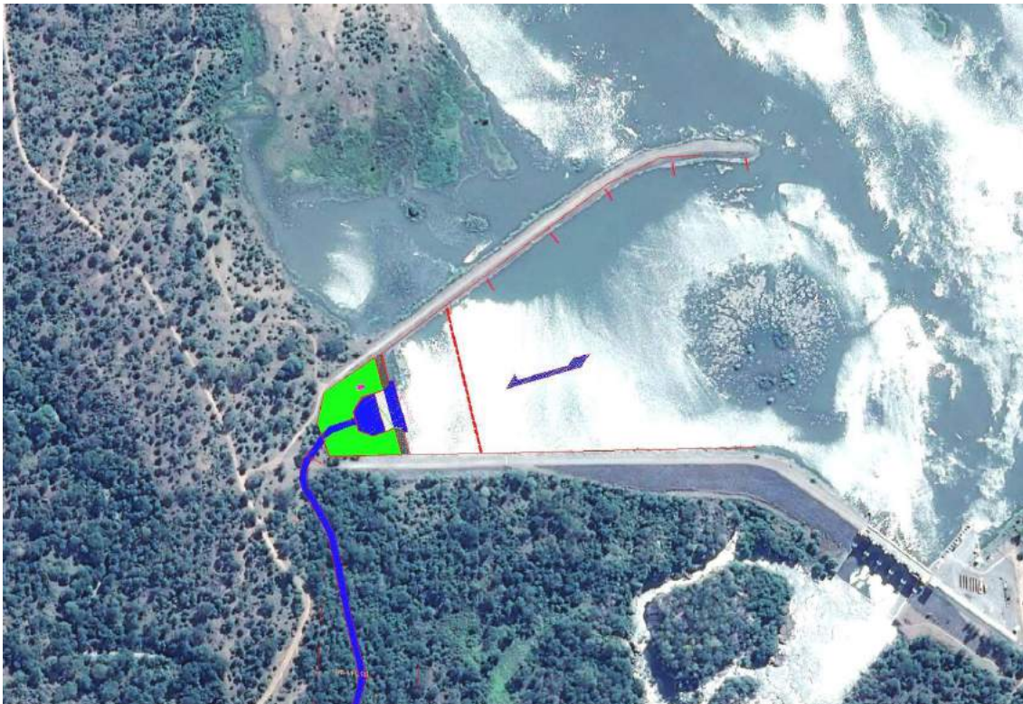
[Figure 2.1-9] Image of intake structure installed at the Site A
