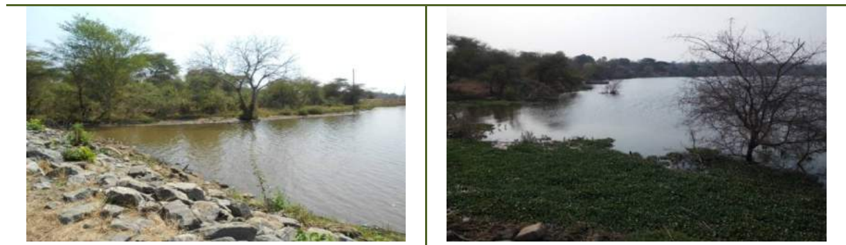
[Figure 2.1-7] Location of Intake Structure at Kapichira Dam Site (Left: Site A, Right: Site B)
