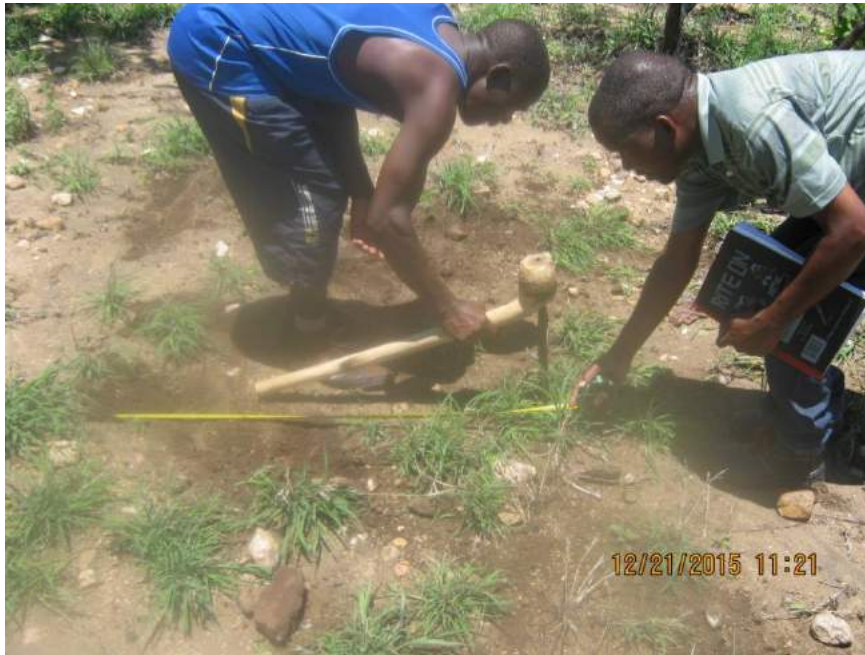
[Figure 2.3-3] Measuring the Surface Dimension of the Pit
