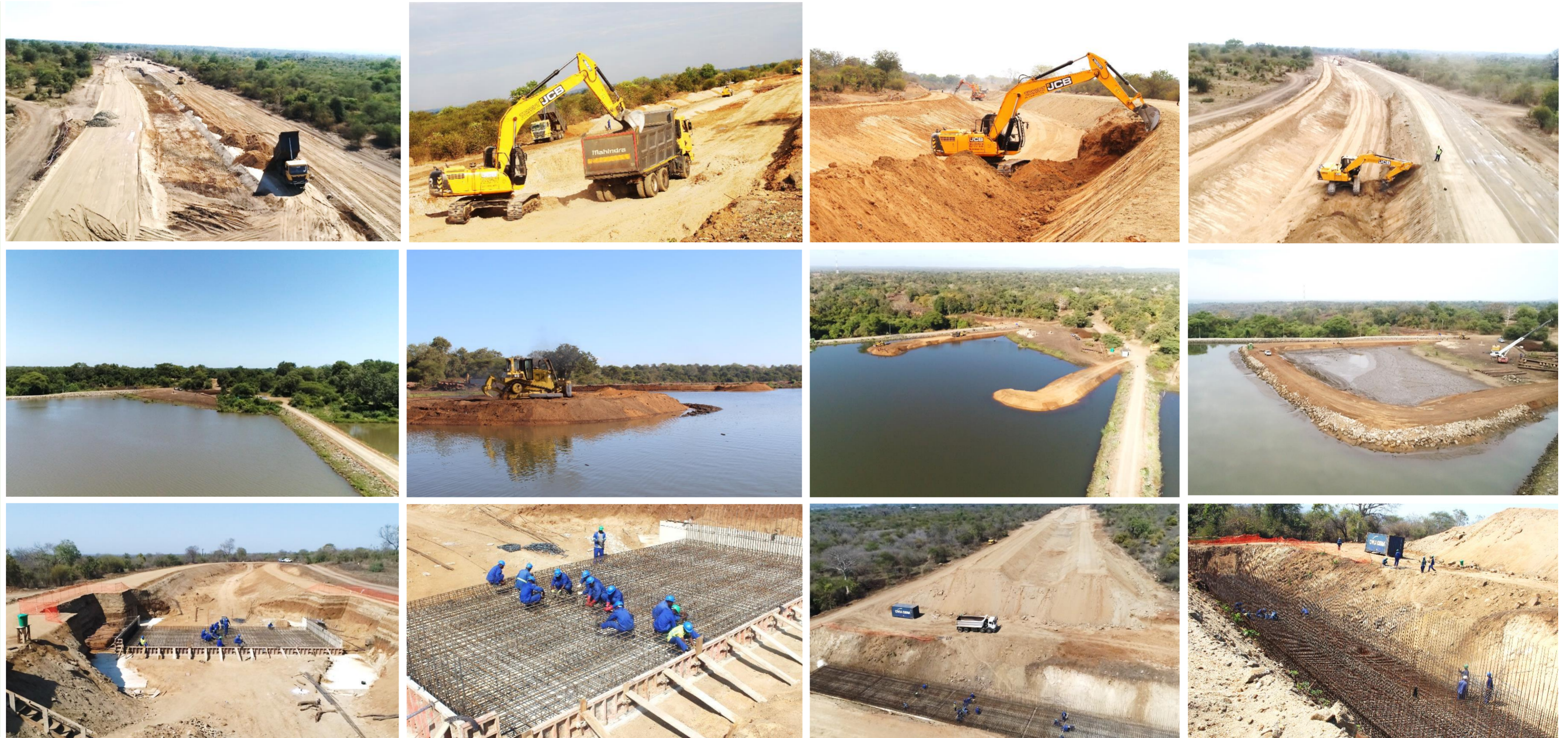
Row 1: (From left-right) - Excavation of the canal route at different stages
