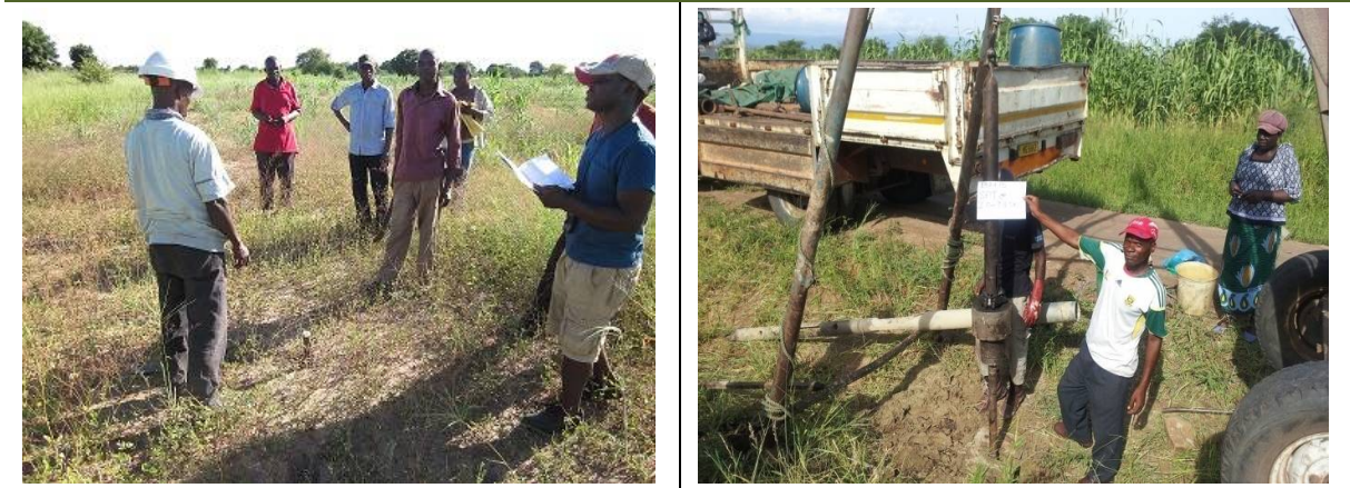
[Figure 2.1] Drilling Point Check(left) and Percussive Drilling & Standard Penetration Test(right)
