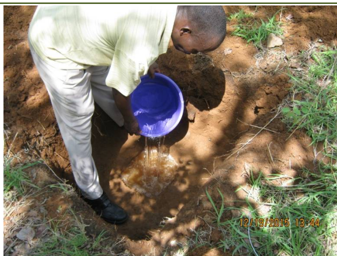
[Figure 2.4] Presoaking the Hole
