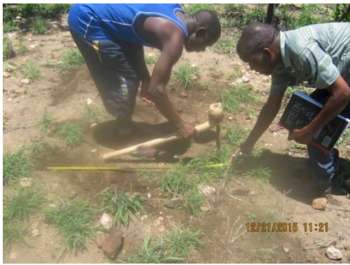
[Figure 2.2] Measuring the Surface Dimension of the Pit (left) and Digging the Pit (right)
