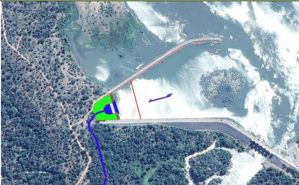
[Figure 6.1-1] Intake Structure in the Kapichira Dam
