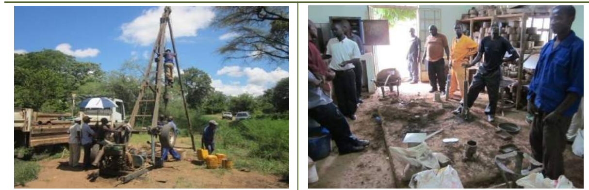
[Figure 8.2-5] Drilling of Borehole (left) and Laboratory Test (right)
