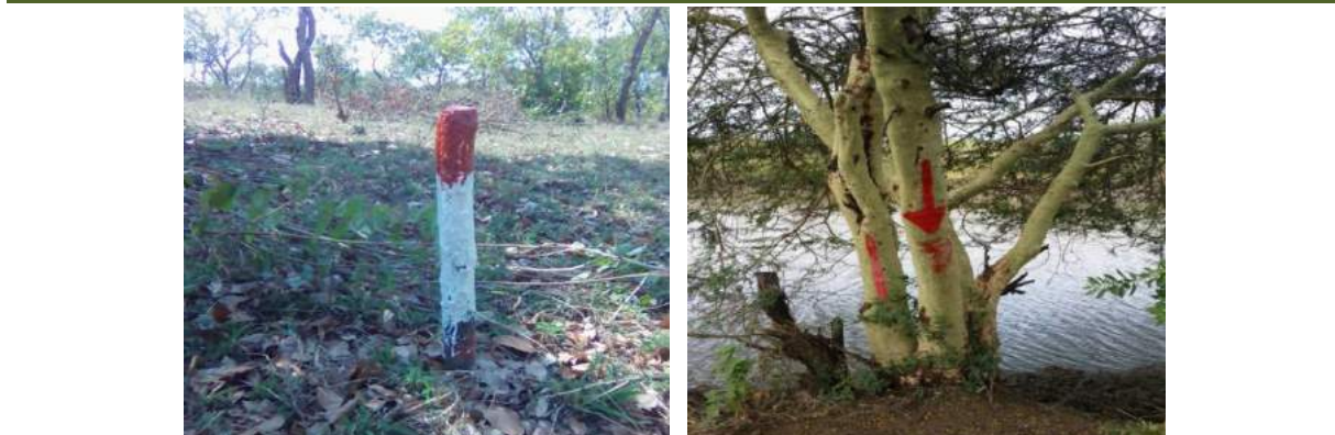
[Figure 8.1-3] Example of Wooden Pegs and Arrow Painted on a Tree along the Canal Centre Line
