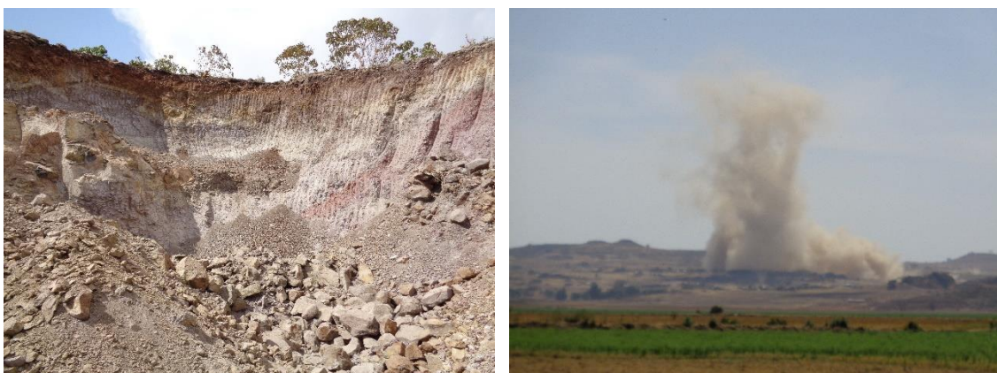
Figure 12 Borrow pit with dangerous steep slopes (left) and typical impact from blasting (right)
