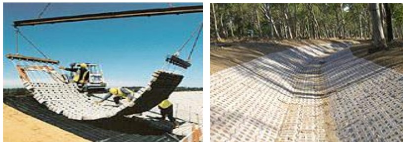
Figure 30 Prefabricated concrete mats (Armorflex ®)
