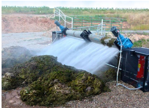
Figure 37 Small scale automatic debris removal screens
