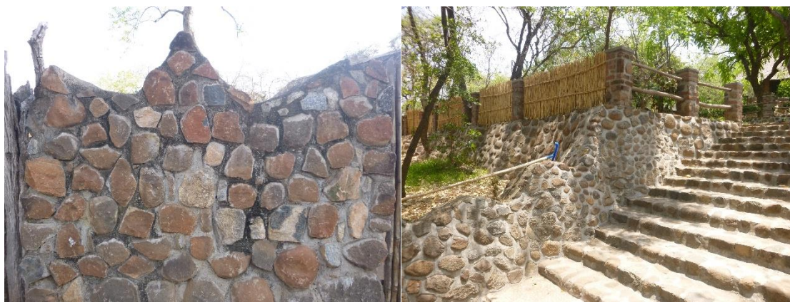
Figure 28 Examples of rock in concrete matrix from MWR and Ng'ona Lodge
