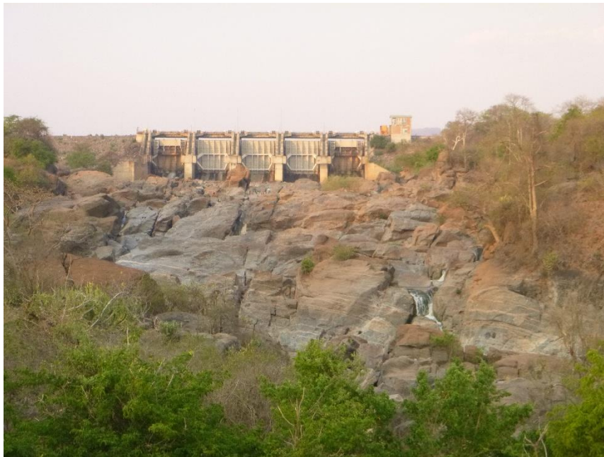
Figure 19 "Invisible" falls at 5m 3 /s (November 2016)
