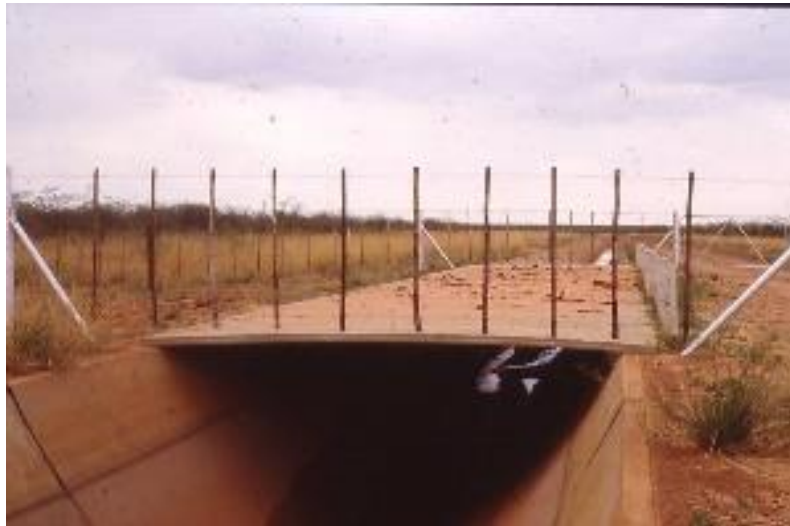
Figure 26 Overpass in Namibia
