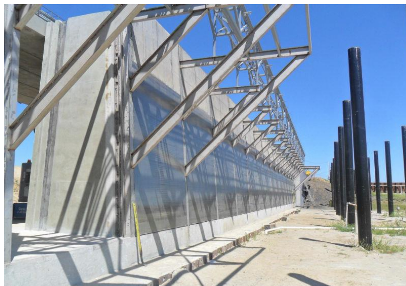
Figure 36 Example of under construction large fish screen for water intake (left)
