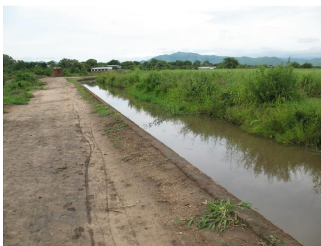
Figure 17 Canal in Kasinthula with still water and aquatic vegetation along the banks
