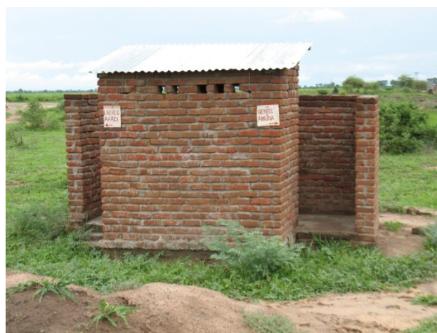
Figure 18 Communal pit latrine in Kasinthula, an elegant but rarely used structure
