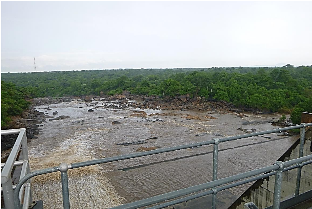
Figure 62 Spillway and environmental flow (left) of 30 m 3 /s
