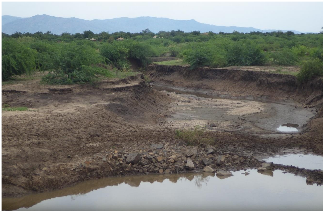
Figure 3 River Bed Digging and Deepening by Erosion in the Namikalango
