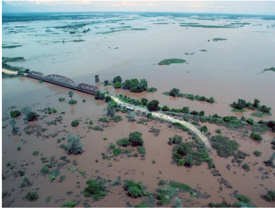
Figure 8 Aerial View of the Shire River and Ruo River at Chiromo Bridge and of the Elephant Marsh Floodplain during the Floods of January 2015
