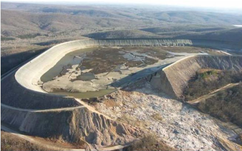
Figure 8.1. Taum Sauk Dam after failure.
