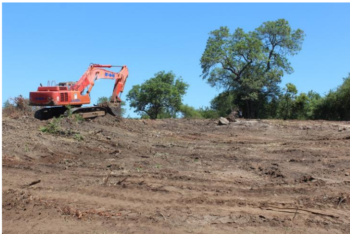
Contractor clearing the site in readiness for construction
